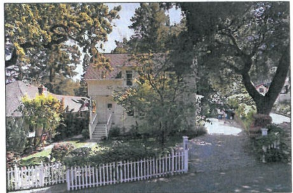
House immediately across Chestnut Avenue
